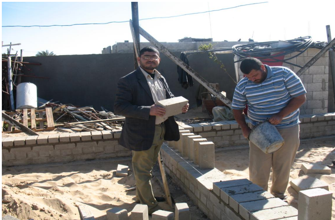
Figure 5.6: Illustrates building the walls with the CSEB (Taken by the researcher, 2011)
