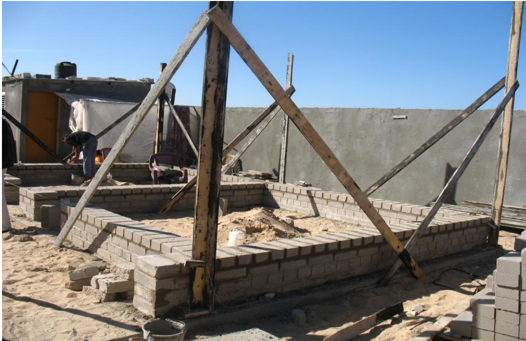
Figure 5.5: Illustrates building the walls with the CSEB (Taken by the researcher, 2011)
