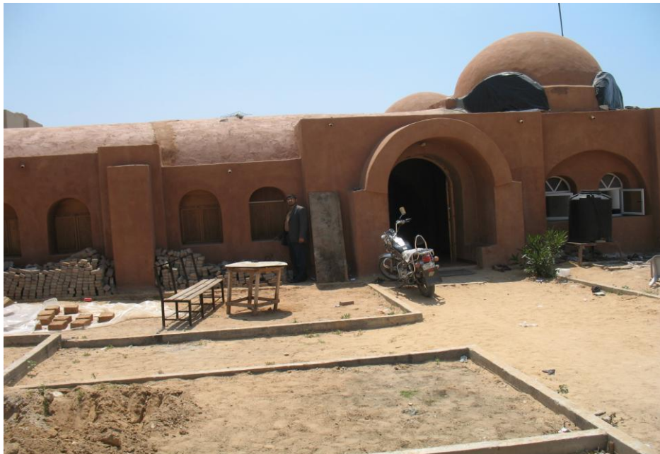
Figure 5.20: Illustrates Police center in Beit Lahiya the walls with the adobe (Taken by the researcher, 2011)
