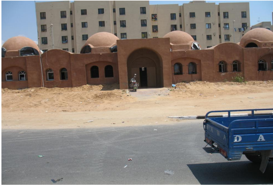
Figure 5.23: The mud building after completion (Ready to be handed to the beneficiaries)
