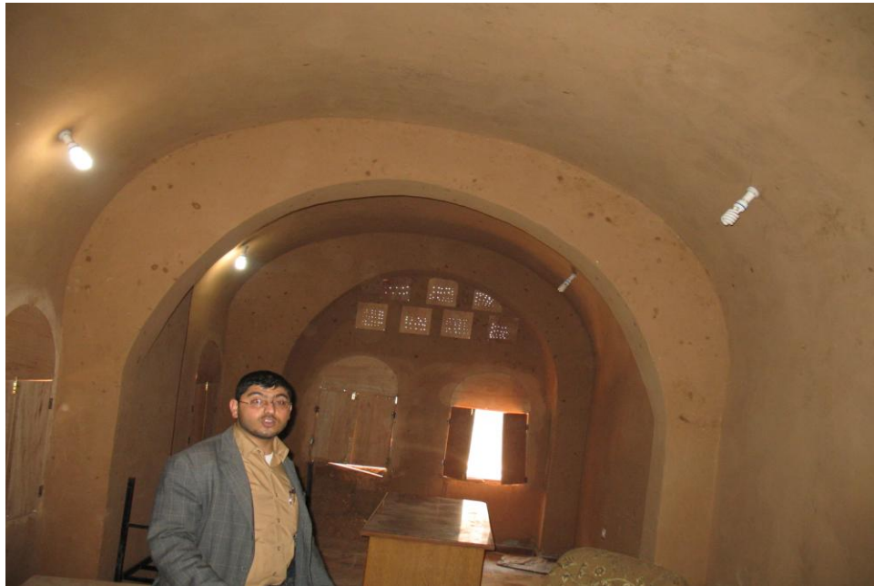
Figure 5.21: Electrical connections in the walls (Taken by the researcher, 2011)
