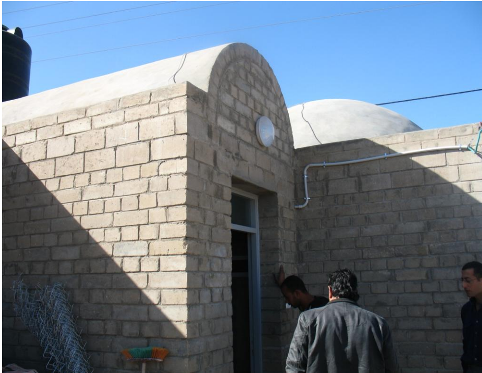
Figure 5.9: The mud building after completion (Ready to be handed to the beneficiaries)
