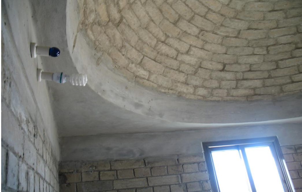
Figure 5.7: Electrical connections in the walls
